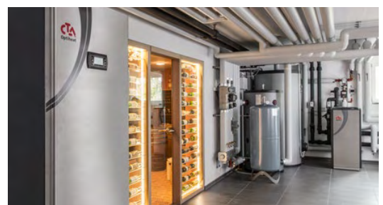
Connection to DHW storage tank, buffer tank and with „free cooling“. The heat pump is connected to geothermal probes.
